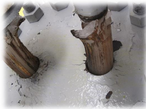
Frozen inlet and outlet water lines
